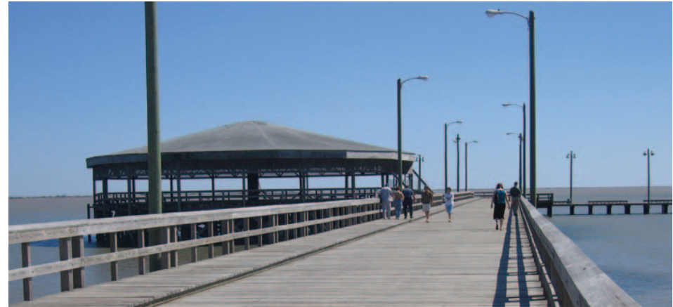
The beautiful Pavillion at the seawall in Palacios
