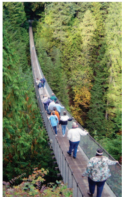
Brave souls take on the Capilano Suspension Bridge near Vancouver, B.C.
